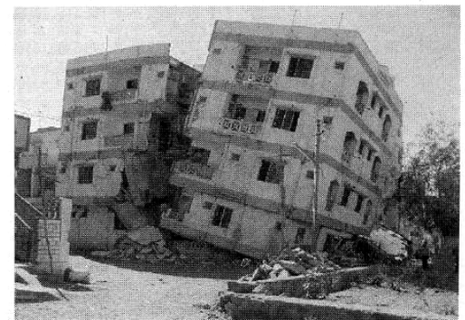
Figure 2: Collapse of the ground storey and vertical splitting of a typical four-storey RC frame building.
