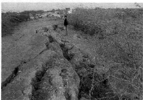
Figure 11: Failure of the upstream slope of the Fatehgad dam.
