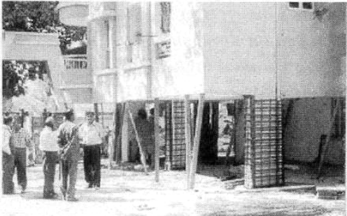
Figure 4: Precariously balanced severely damaged RC frame building with open ground storey in Ahmedabad.
