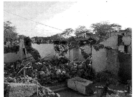
Figure 1: Total collapse of traditional houses in random rubble stone masonry with mud mortar at Maliya village.
