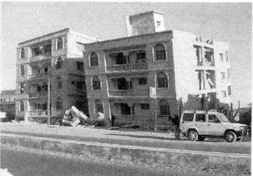
Figure 5: Ground storey collapse of a 4-storey building with open ground storey at Bhuj.
