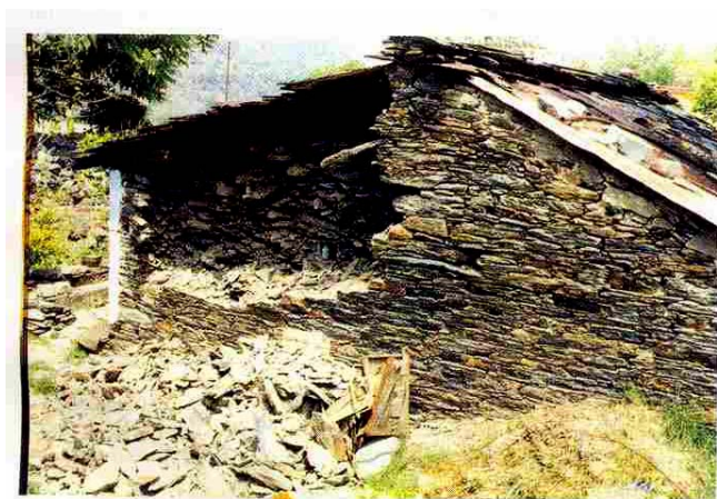
Figure 7. Collapse of one of the wythes in a traditional house in slate wafer masonry.
