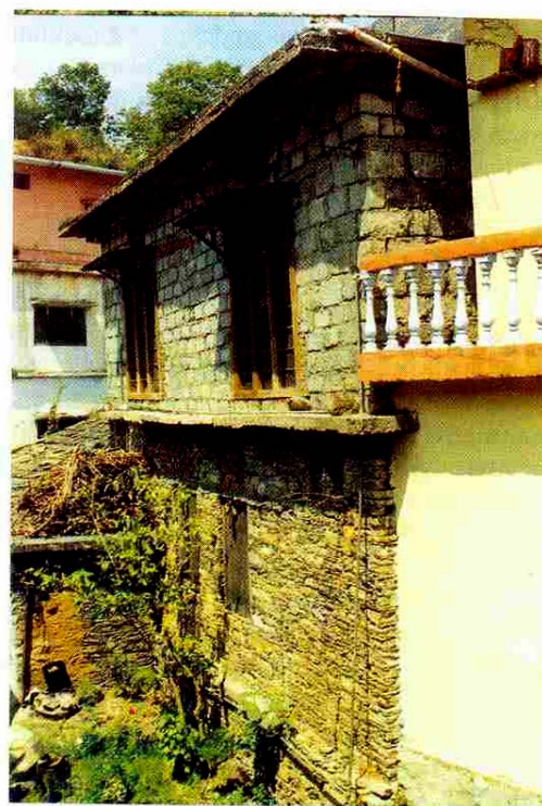
Figure 8. Two-storey house at Pipalkoti showing no damage. The ground storey is in slate wafer masonry, upper storey in concrete block masonry has been added later. Both storeys have RC lintel band.
