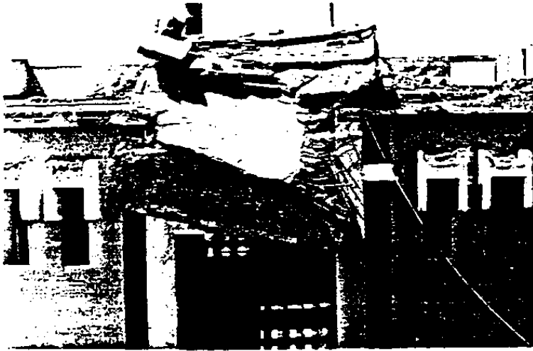
Figure 3: Close-up view of the mummy collapse in the Department of Telecom housing colony.
