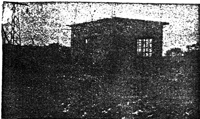
FIG. (2) A R.C. FRAME BUILDING IN SILIGURI WITH "LINTEL BAND"
