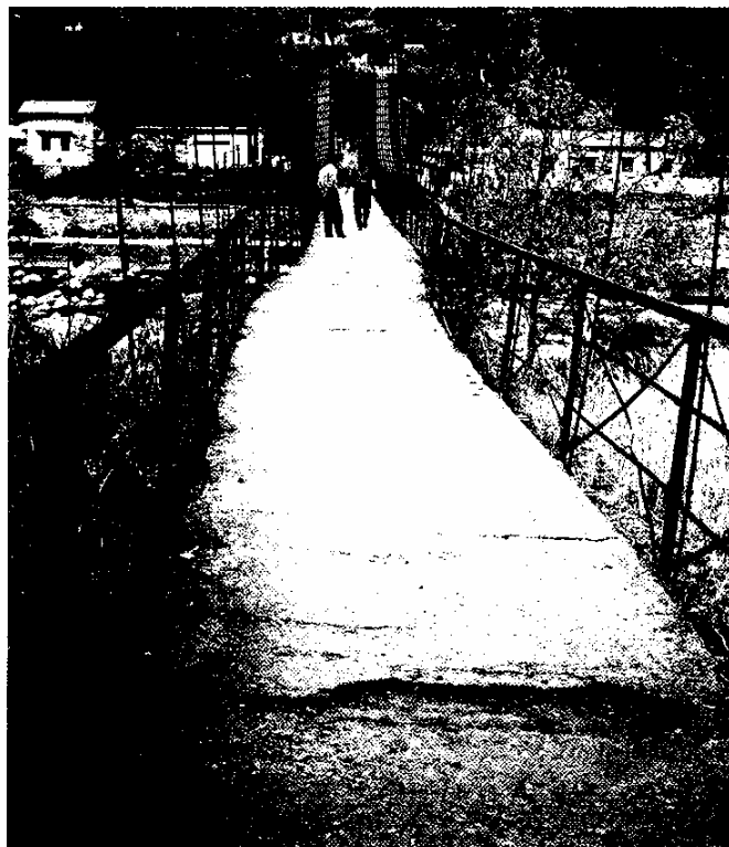
Figure 10: Lateral buckling of the deck of a suspension bridge at Bairagna.
