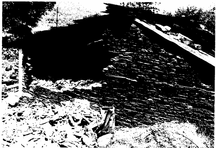
Figure 5: Collapse of one of the wythes in a traditional house in slate wafer masonry.
