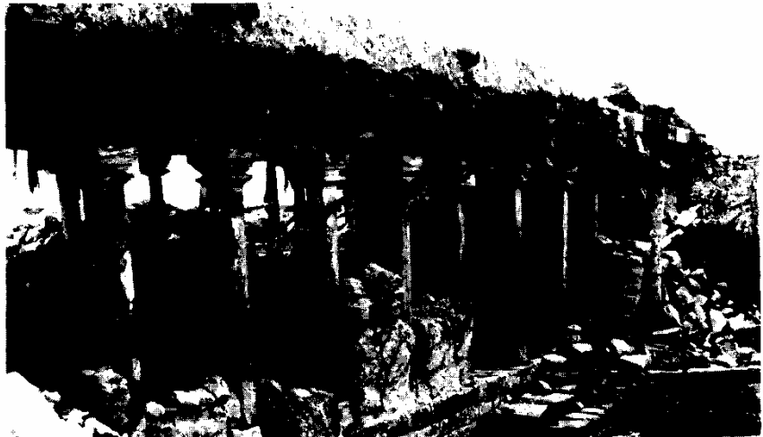
Figure 5 - In some buildings, the traditional heavy clay roof was supported on a frame of wood posts and beams. In most cases, the timber columns continued to hold the roof together while the walls collapsed, generally outwards from the timber frame, saving the lives of many occupants.
