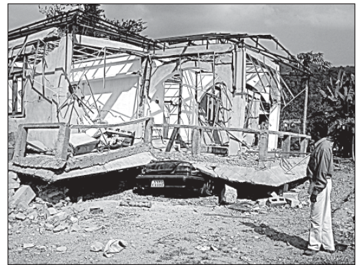
Fig 3 Collapse of a stilt plus one-storey house in reinforced concrete near Port Blair (Photo: Sudhir K. Jain)
