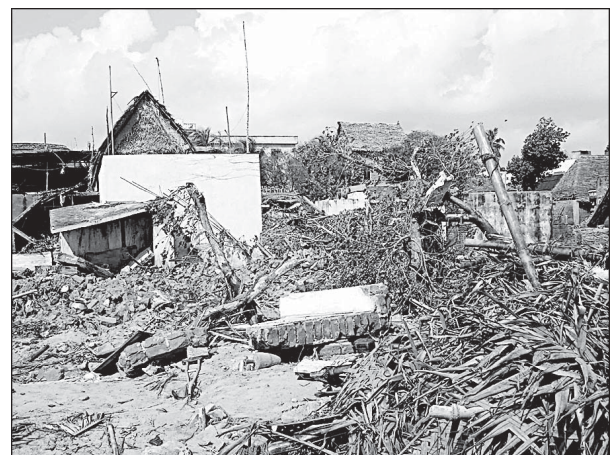
Fig 8 Ravaged houses at Nagapattinam due to poor construction (Photo: Alpa Sheth)
