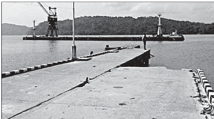
Fig 7 Collapse of the 80-m segment of the approach to Great Nicobar island jetty at Cambell Bay. This has adversely affected the relief work (Photo: CVR Murty )
