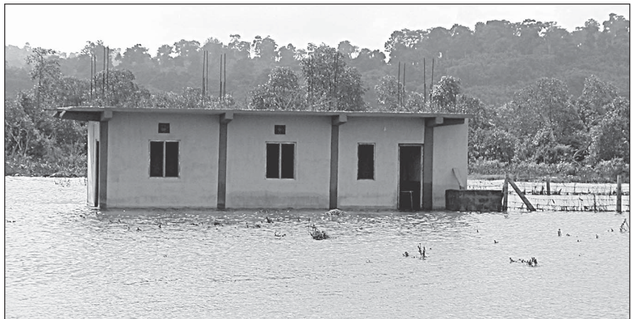
Fig 1 Sea water level at Port Blair with respect to land has gone up by about 1 m. Hence many areas are now flooded during high tide (Photo: Sudhir K Jain)
