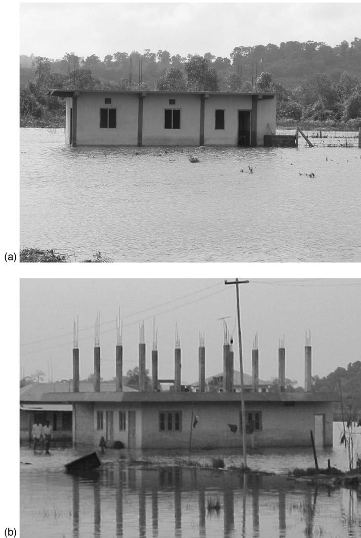
**Figure 13.** Inundated single-story houses such as these suggest that the seawater level has gone up by about 1.0 m with respect to land in the Sippyghat area near Port Blair. Many areas are now flooded permanently because of land subsidence (photos: S. Jain and C. Murty).
