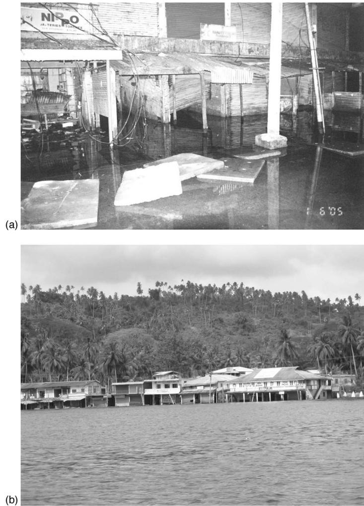
**Figure 12.** Subsidence caused the inundation of land in the bazaar area of Bamboo Flat (photos: J. Malik and D. Rai).
