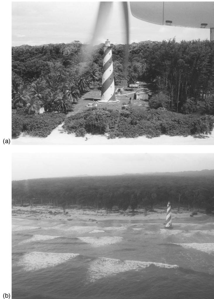
**Figure 8.** (a) The lighthouse tower at Indira Point in Great Nicobar Island before the 26 December earthquake. The tower is surrounded by lavish green grass, residences are at the base, and a sandy beach is in the foreground. (b) Flooding of the lighthouse base because of land subsidence. The submergence of  $\sim 3$  m was caused by the 26 December earthquake (photos: R. Makwana).
