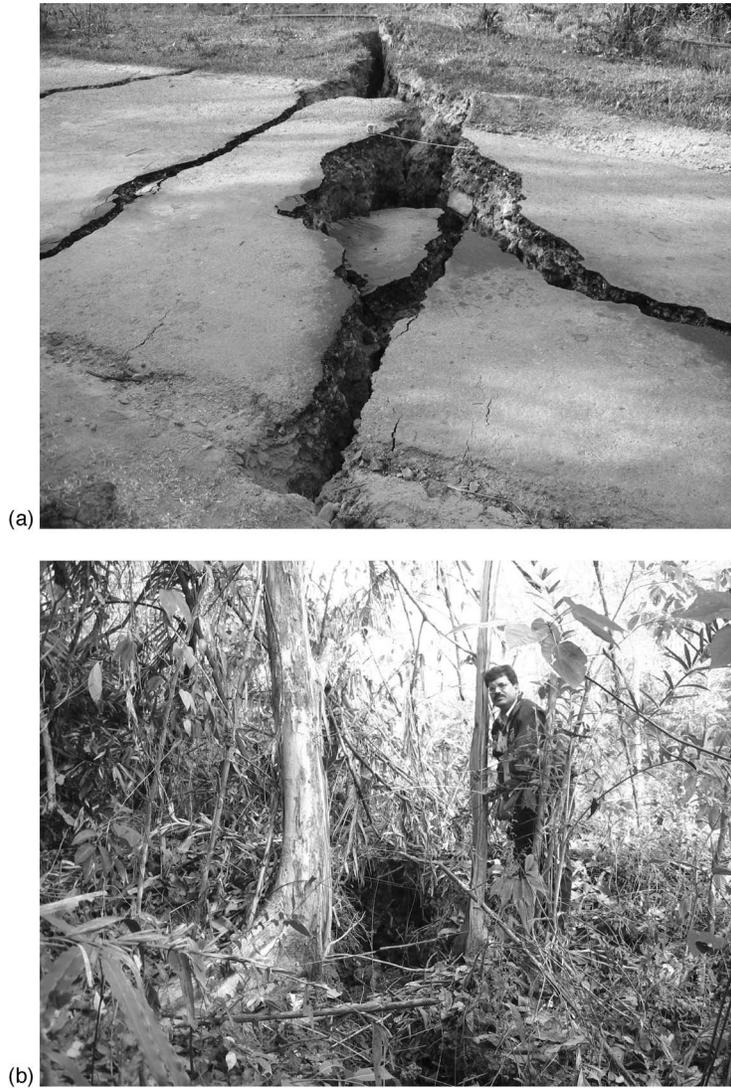
**Figure 19.** Ground deformation at Jarawa Creek at Baratang Island near Middle Andaman Island. (a) Damage to a road connecting Baratang Island and Baludera Beach (photo: D. Rai). (b) Splitting of a tree trunk because of a ground rupture  $\sim 1.2$  m wide (photo: G. Mondal).
