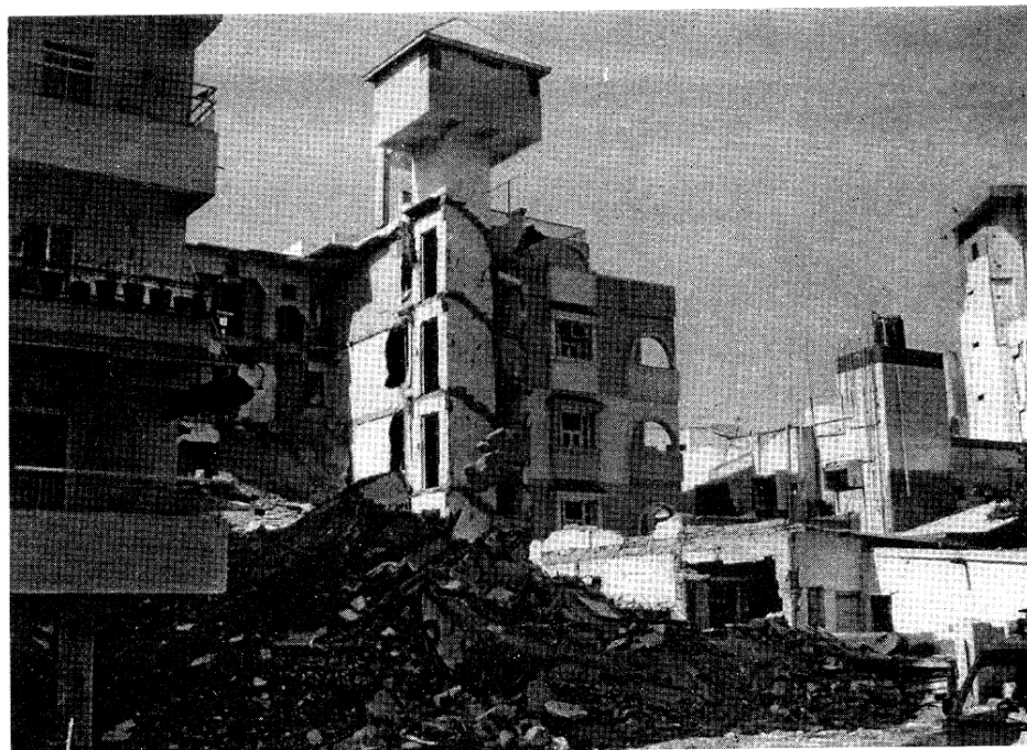
Fig. 5 Collapse of a 4-storey RC building in Ahmedabad due to inadequate connection between the RC elevator core and the building.
