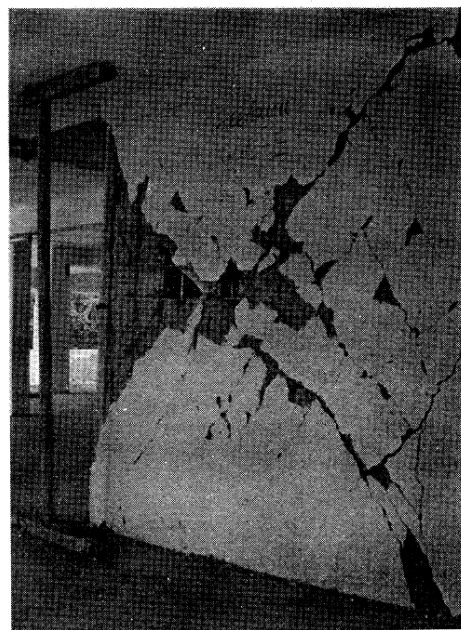
Fig. 4 Severely damaged RC elevator core of a 5-storey building in Ahmedabad
