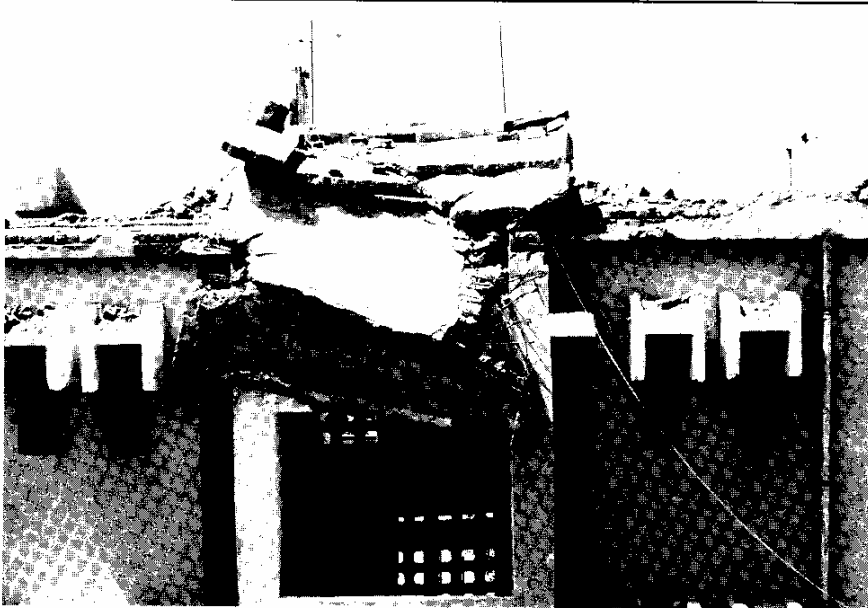
Figure 5 - Many staircase towers, called "mumty," which project about 2 m above the surrounding construction in masonry houses, collapsed.
