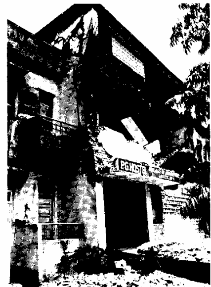
Figure 4 - Load-bearing brick masonry structures on the campus of Jawaharlal Nehru Agricultural University in Jabalpur were badly damaged.
