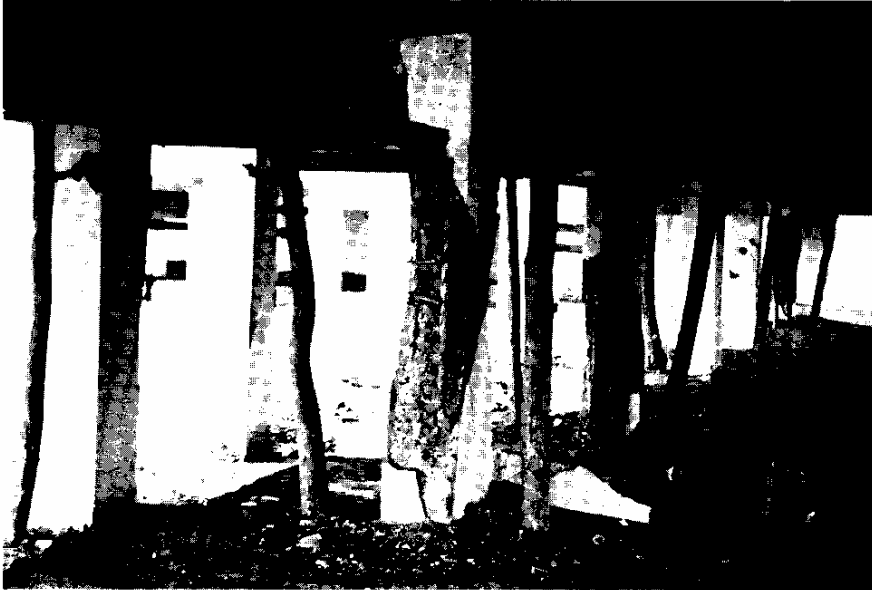
Figure 7 - Built on piles and stilt columns on the site of a previous pond, the new, still unoccupied Youth Hostel in Jabalpur suffered serious damage to its stilt columns.
