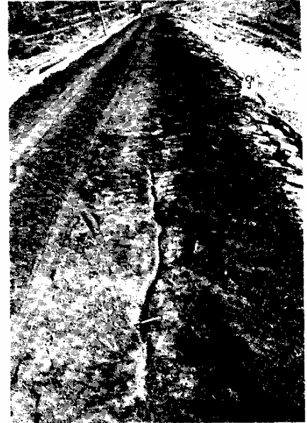
Figure 10 - Longitudinal cracks appeared along the crest and downstream face of several earthen dams.
