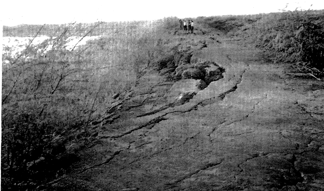
Figure 5: Liquefaction induced failure of the Fatehgarh dam.
