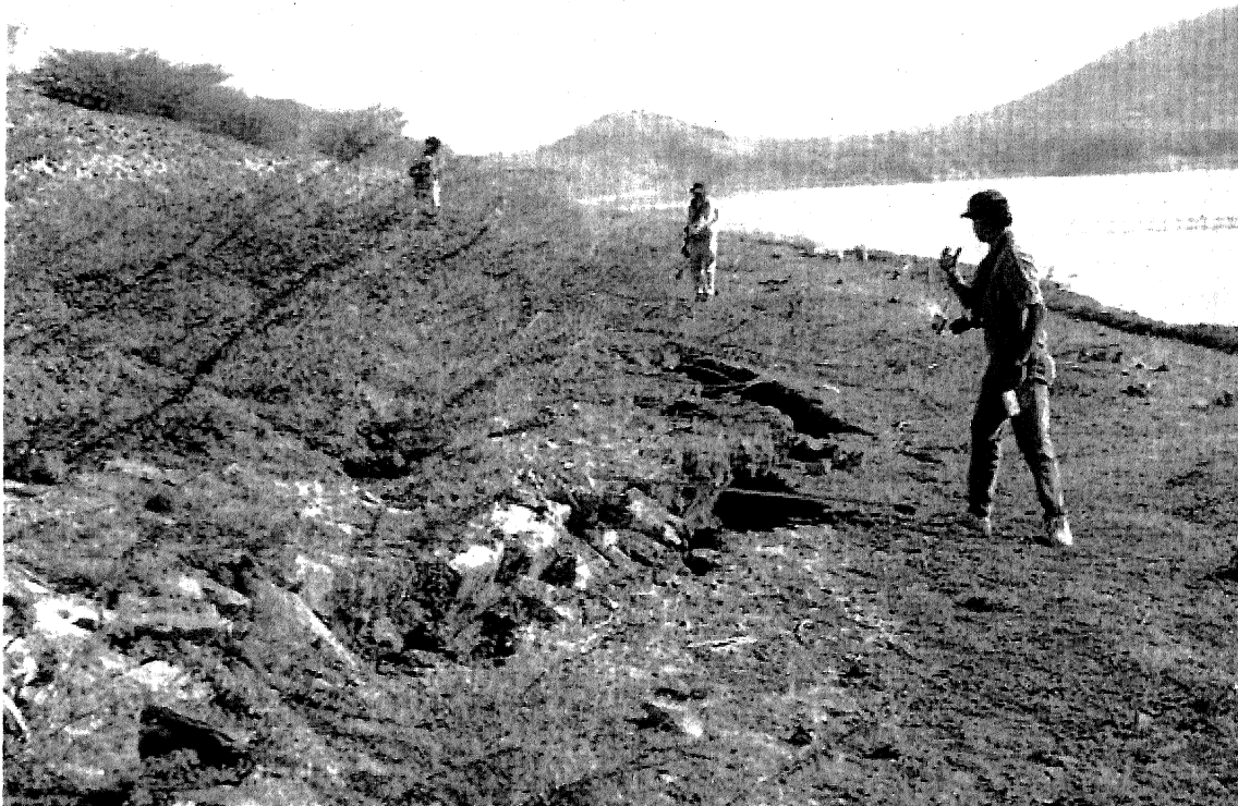
Figure 9: Massive crack near the upstream toe of the Kashwati dam.
