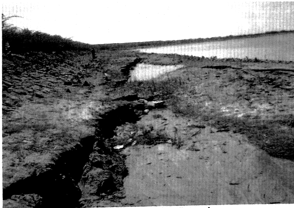
Figure 8: Lateral spreading near the upstream toe of the Tappar dam.
