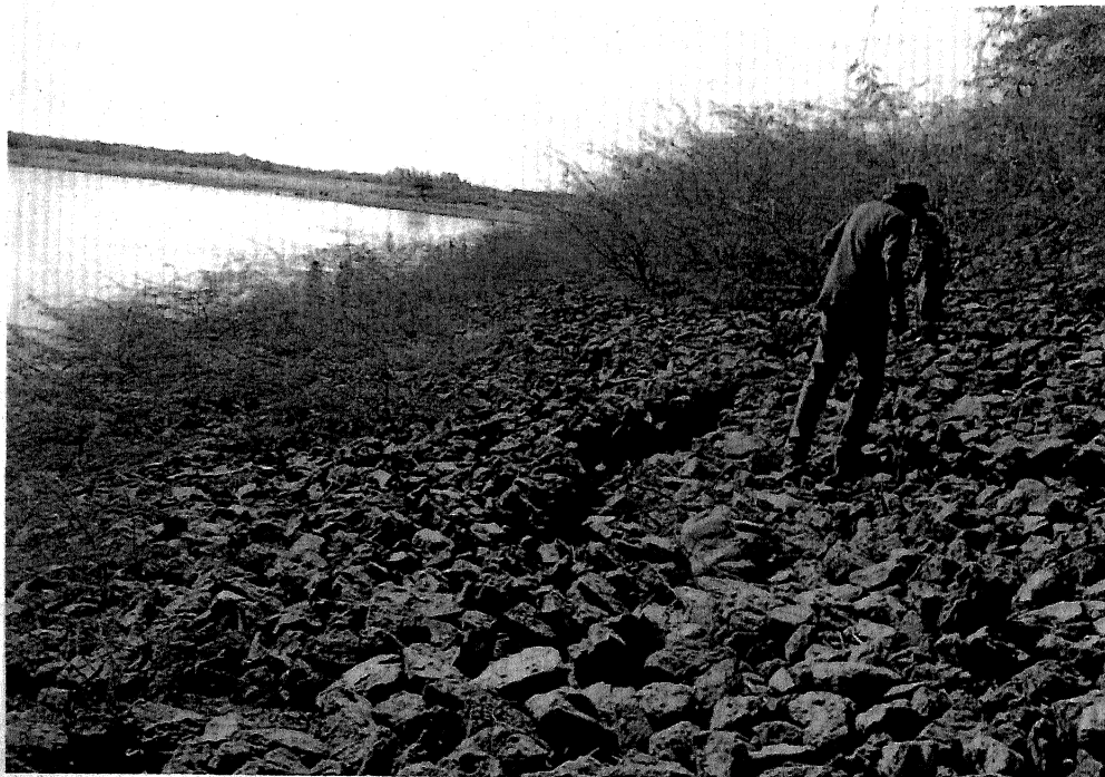
Figure 7: Lateral spreading owing to liquefaction of the upstream toe of the Suvi dam.
