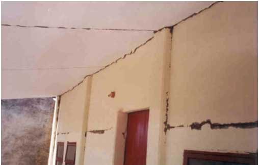
Figure 14-11. Type C damage — minor dislocation of roof planks.
