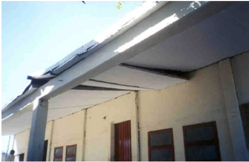
Figure 14-10. Type B damage — roof planks slipped.
