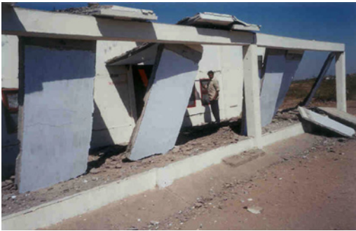
Figure 14-9. Type A damage — major damage to structure.
